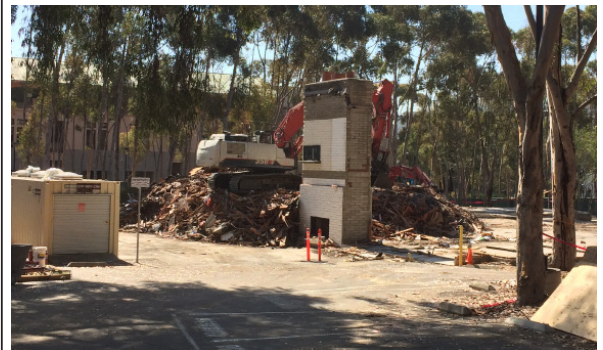
By early July 2017 only the IC's chimney remained standing
