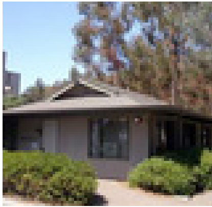
Bldg. 214, the new home of the Friends Resale Shop, as well as the Friends Office. Located off Library Walk and the north side of Rupertus Way. It is adjacent to Bldg. 215 that houses the Office of the Dean of the International Center.
