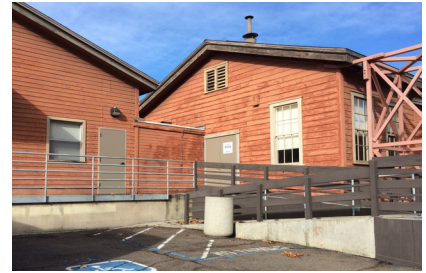
Bldg. UC 409 is located at intersection of Rupertus Lane and Russell Lane, across from the Visual Arts building, and near the Gilman Parking Structure
